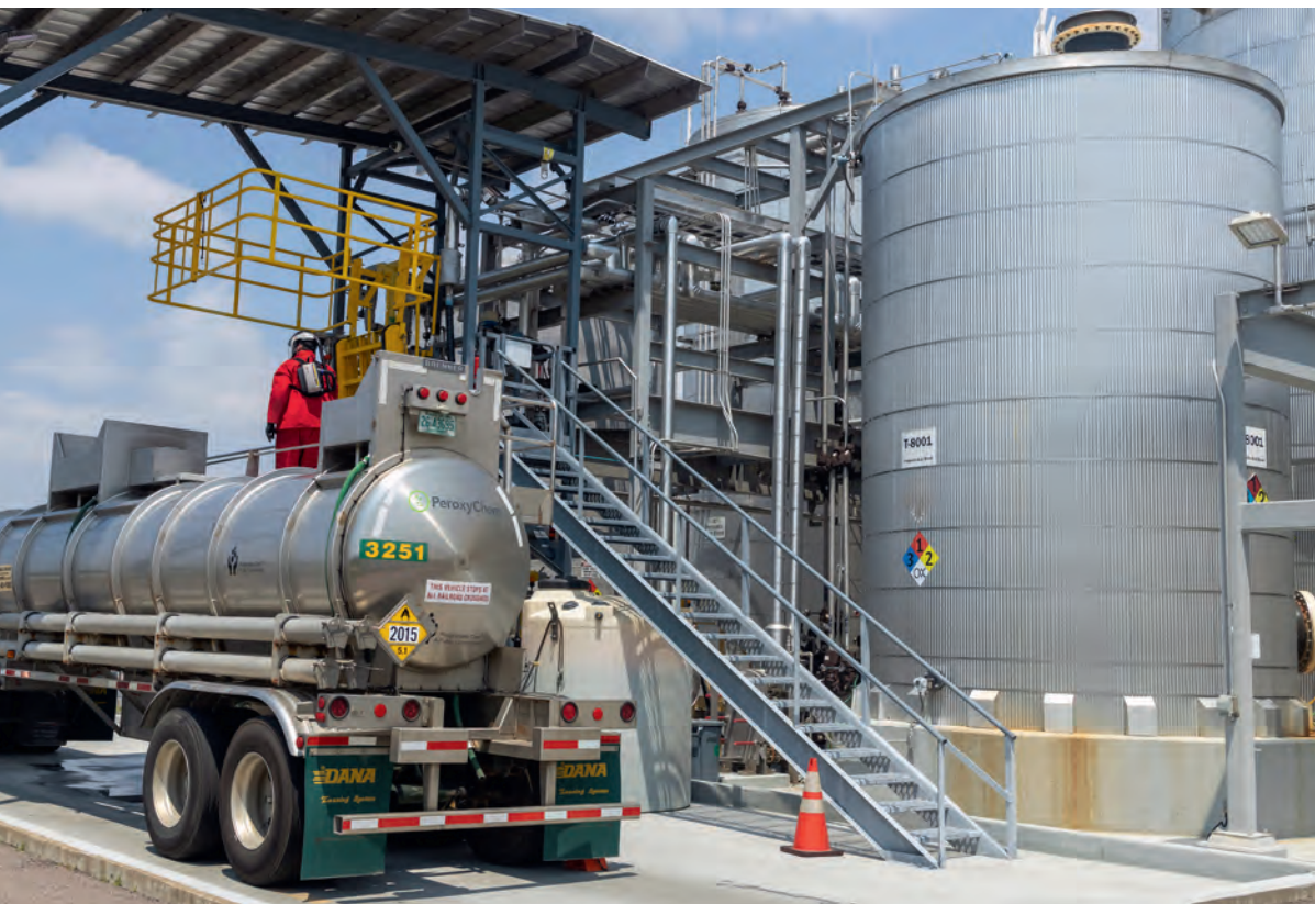
A worker prepares to offload hydrogen peroxide for the production of the disinfectant peracetic acid at Evonik's Wolf River plant.
